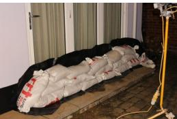
Sackmaker fill our sandbags with approximately 14 kilos of washed Granite Sand.
