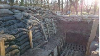
Hessian Sandbags eventually rot away so are ideal to fill with sand /cement mix and leave to form a wall or fill with soil & seeds to create "living roofs" and other structures.
