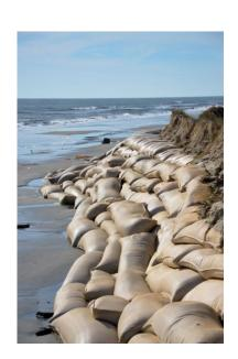
Variable amounts of UV & weather exposure mean predicting Sandbag longevity is not an exact science, so we field test ours in real applications. As a rough UK guide our Standard White WPP Sandbags last around 6 months while heavy duty Reusable Sandbags take around 2 years before starting to break down.
